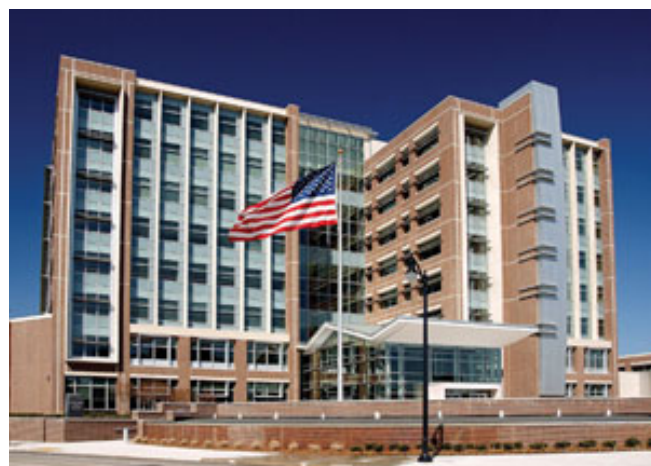
Photo courtesy of Opus South Corp., Atlanta The completed Birmingham Social Security Administration Center has achieved LEED® Silver Certification.
