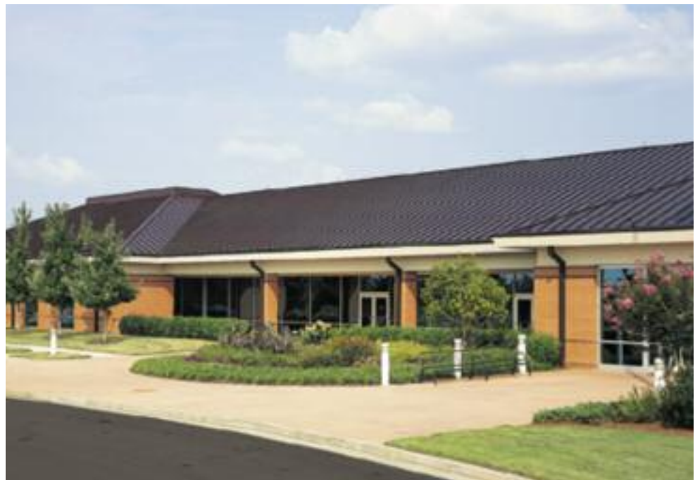
Bottom Photo: Cingular Wireless Customer Service Center Cedartown, GA Distributor: CRS - Atlanta Architect: Rosser International Roofing Contractor: West Georgia Roofing Custom Color: Raisin
