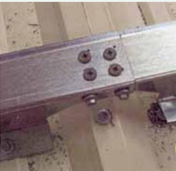
threads/inch pancake heads, denoted #12-11 x 1" S.D. Pancake Head; plus 2 -#12-14 x 1- $\frac{1}{4}$ " Tek-3. At the point where the Roof Huggers lap 4 pancake heads are installed in the top flange and the 2 Tek fasteners in the vertical flange.
