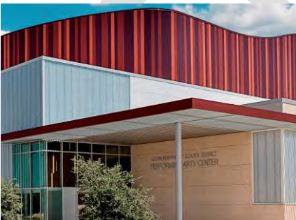
Three colors of wall panels create the mosaic pattern seen on this fine arts facility in Texas.
