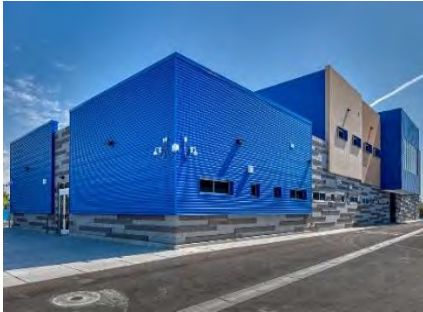
Bright blue wall panels with horizontal ribs make a bold statement on this school in Nevada.
