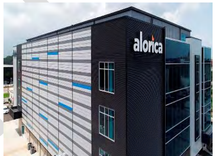
Metal wall panels in multiple colors create visual interest to multi-story structures like this office building.
