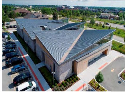
This health care facility in Illinois features three butterfly-like roof systems using standing seam architectural metal roof panels.
