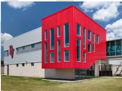
Three shades of red were chosen to create this bright mosaic pattern on the corner of this vo-tech high school in Texas.
