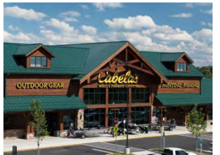
This Cabela's store features a standing seam metal roof system in custom green color to complete the log cabin aesthetic architects envisioned.
