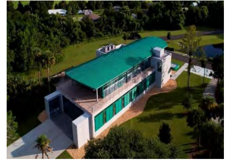
Metal roofs can be curved to add drama to a roof, such as the custom green roof panels seen on this aquatic center on a college campus in Florida.
